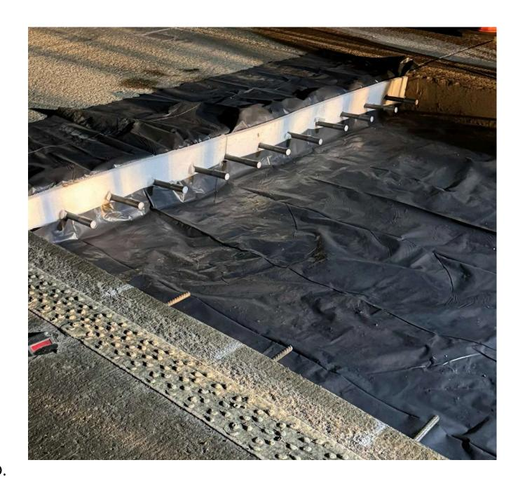
Once they've finished removing the damaged concrete, the crew begins to prep the area with a waterproof membrane and steel tie bars before pouring the fresh concrete.
