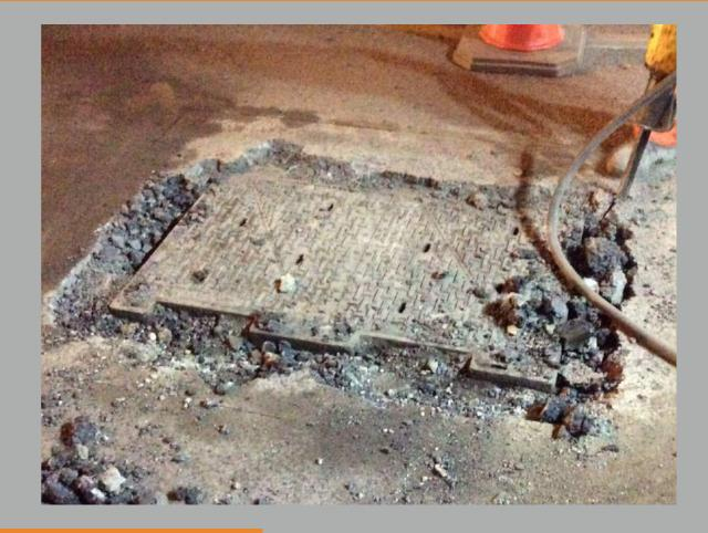
"LMS have carried out the replacement of a large proportion of the carriageway ironwork assets, enabling the ironwork replacement works to be completed successfully and the road opened to trafficking every morning." Balfour Beatty Mott Macdonald, Spokesman.
